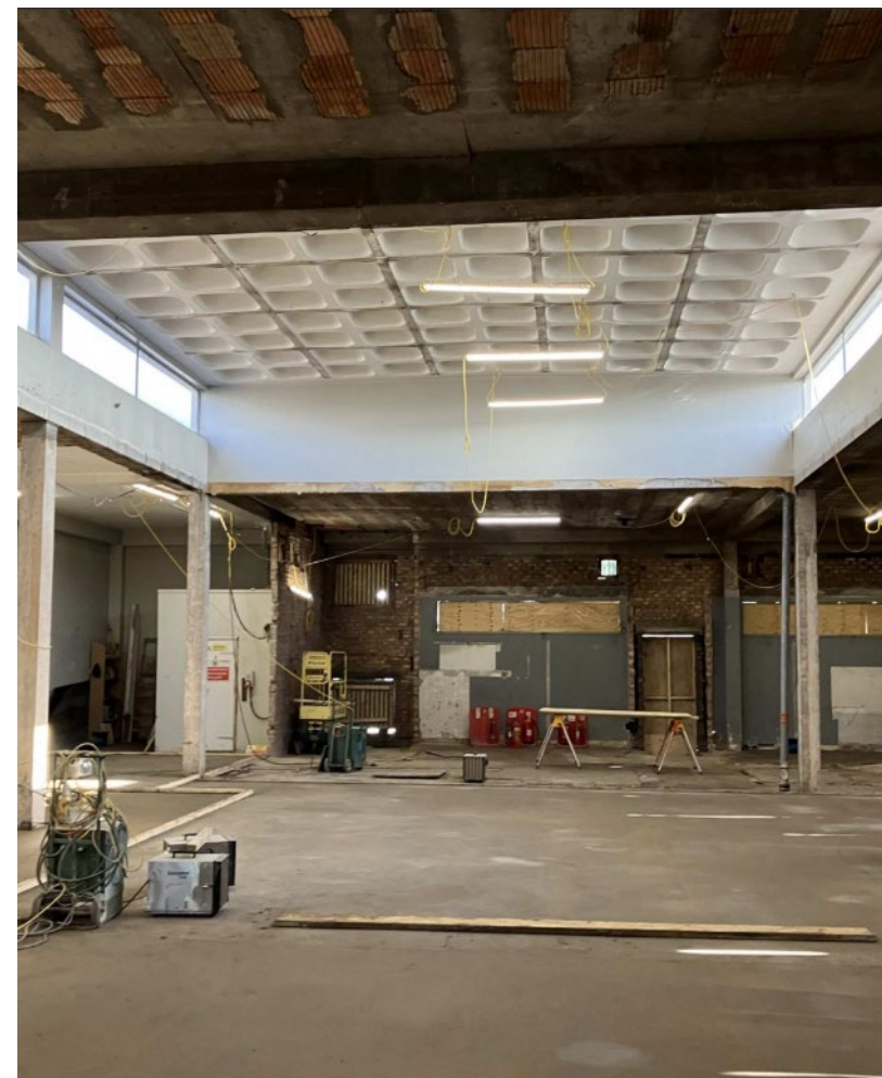
Retrofit 2026 – sustainability in practice in creating the Manchester City Women’s HQ – incorporating a former bank building.
